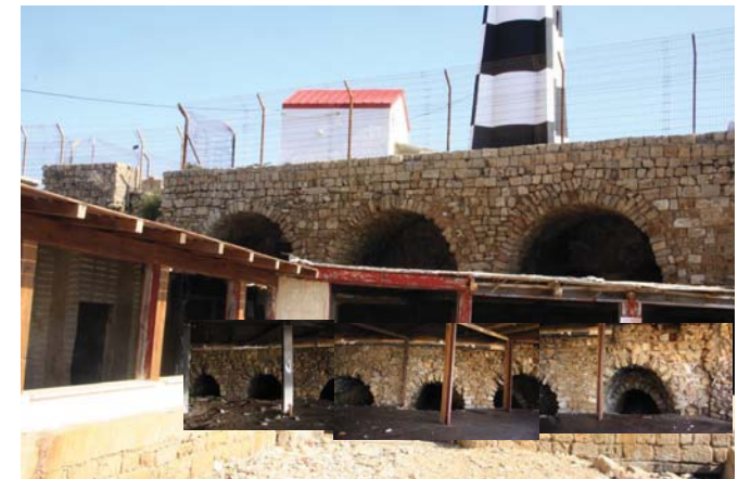
similar two storey vaulted structure beneath the light house (intergrated photos)
