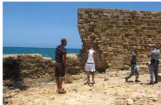
vandalism: burning garbage
