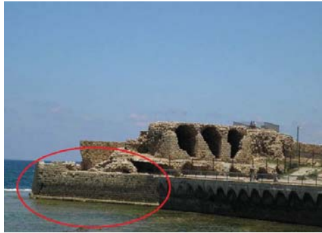
Figure 14: The lagoon wall of the Structure built either during the last year of the British Mandate or during the 1960s reconstruction of the lagoon reinforcement wall.
