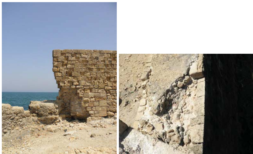
Figure 5: The first picture illustrates the difference in building technology between the sea and the lagoon walls; the second picture illustrates the Ottoman technology of wall construction.
