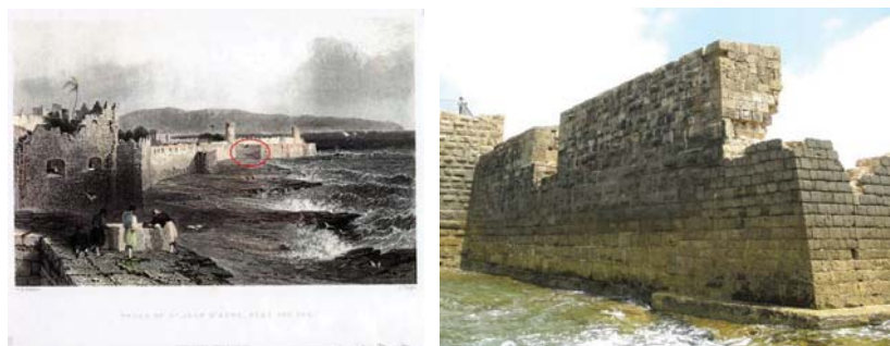
Figure 8: On the left: W. H. Bartlett. A View to the Western Walls of Acre from the North, 1836. On the right: the present condition of the wall circled on Bartlett's engraving.
